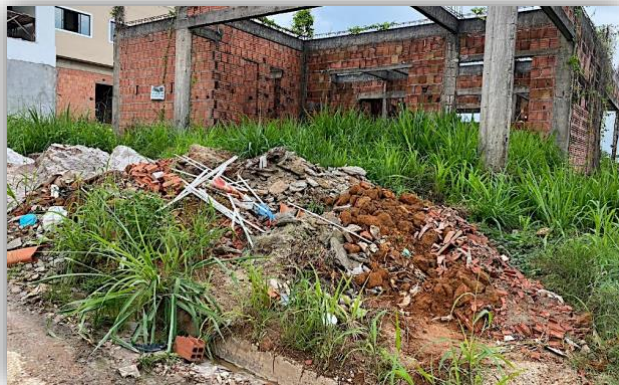
Figure 3.1. RCC waste in the urban core.
