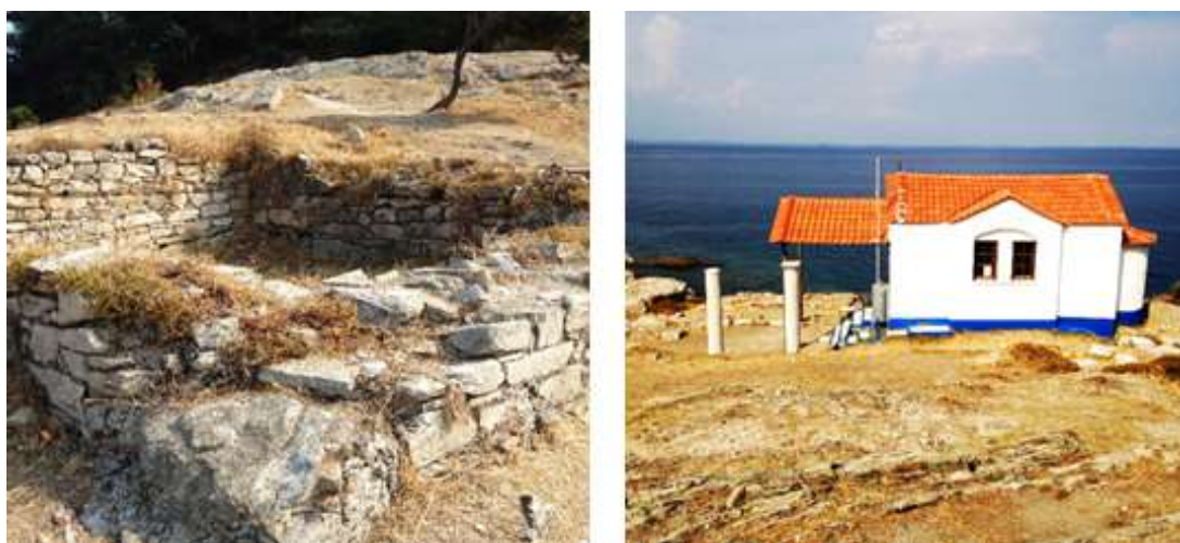
Fig.8a - Structure of a 6th century B.C. terrace. Personal archive, 2015.
