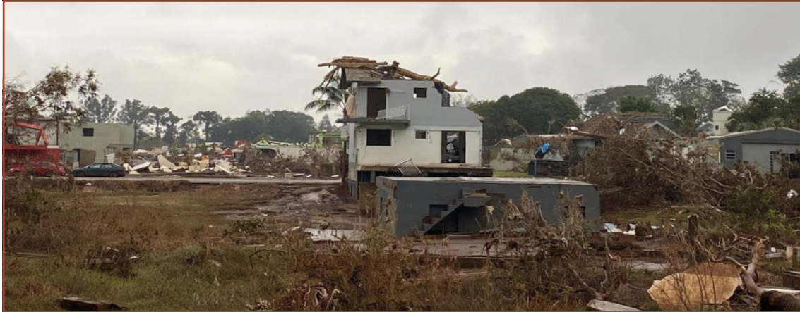
Figure 7 – Current partial view of Arroio do Meio
