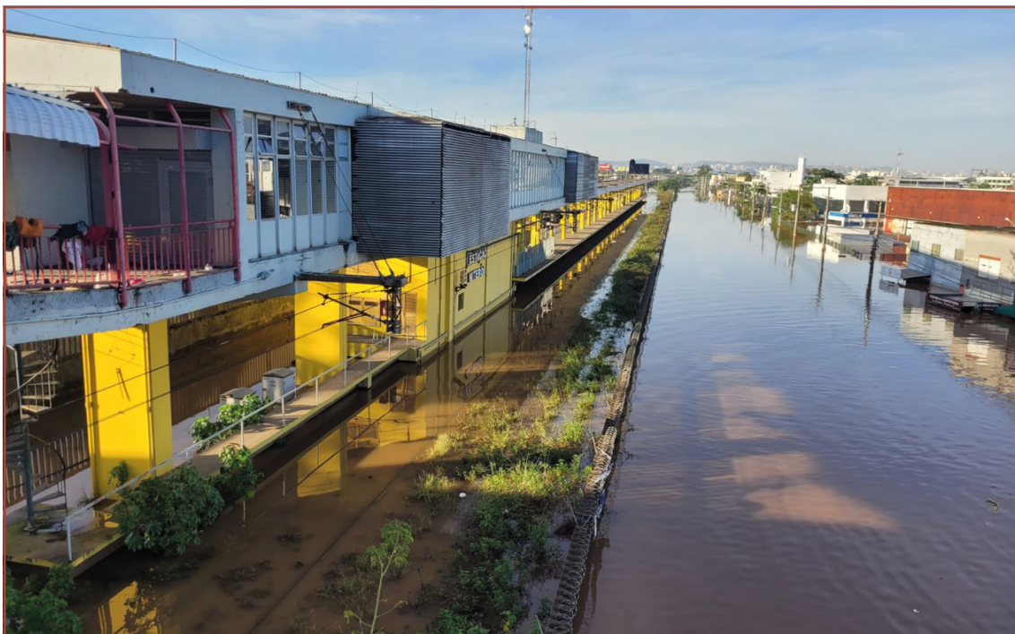
Figure 12 – Niterói Station of Trensurb Metro flooded in Canoas
