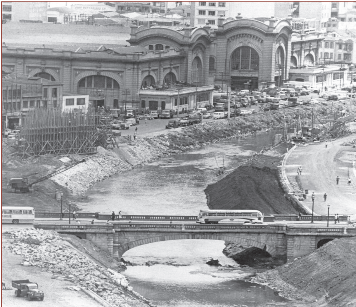
Figure 8 – Channeling works in the Tamanduateí River in the Municipal Market area in 1969
