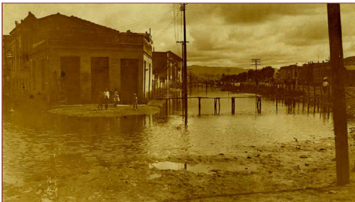
Figure 7 – Flooding of the Tamanduateí River at Cantareira Street (1930s)
